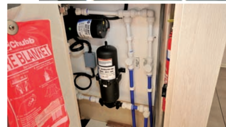
Easily understood plumbing, with fresh water pressure pumps grouped together in a galley locker. I liked the thermo-engraved labeling
